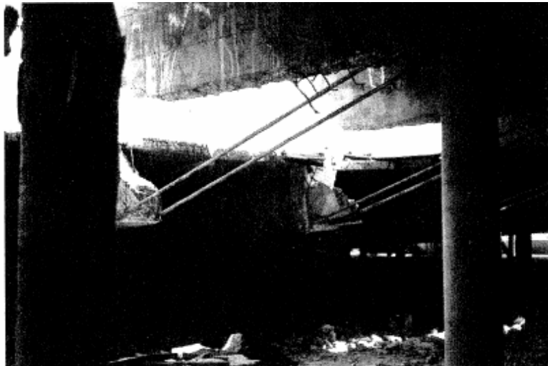
Figure 2-14 Failed roof beam demonstrating continuity of bottom steel [Degenkolb, 1987]
