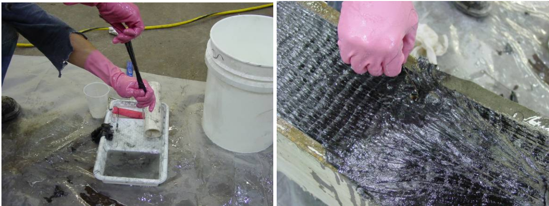
Figure 3-39 Saturating anchor and making hole in CFRP sheet to insert anchor
