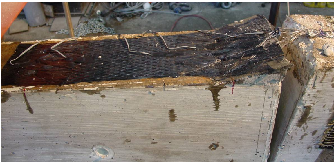
After Testing: Failure by FRP fracture
