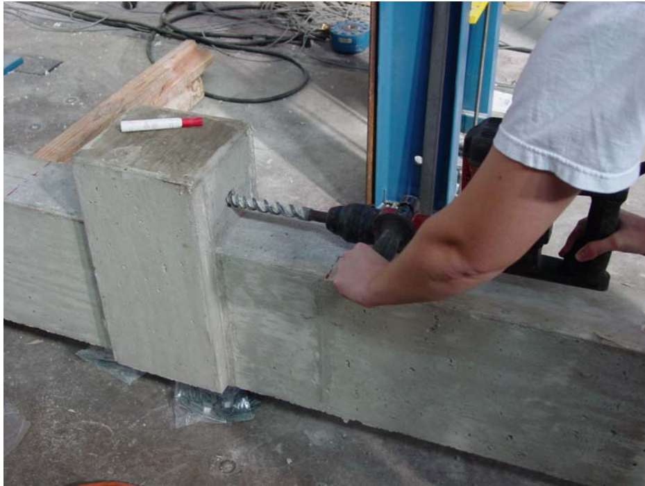
Figure 5-22 Drilling hole through column
