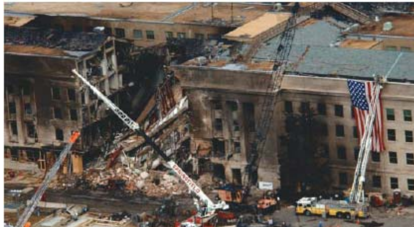
Figure 2-9 Collapse of Pentagon building [Mlakar et al., 2003]
