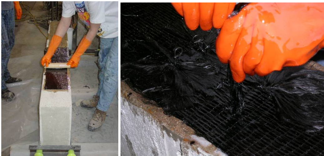
Figure 3-37 Removing air bubbles from CFRP sheet and applying CFRP anchors
