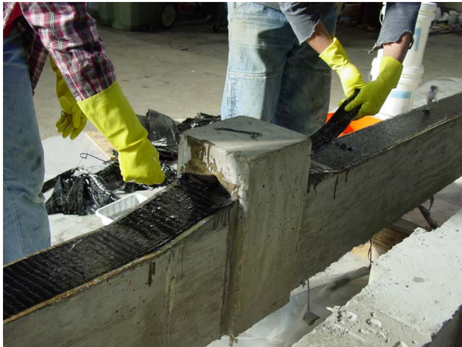
Figure 5-23 Pulling CFRP through hole in column
