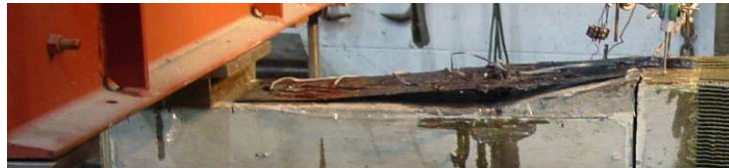
Fracture first row of anchors
