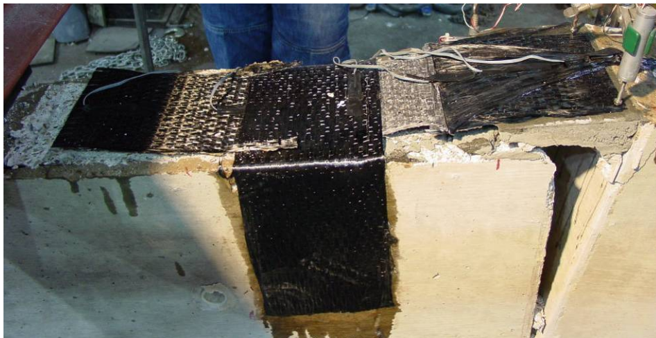
After Testing: Failure by FRP sheet slipping under U-wrap
