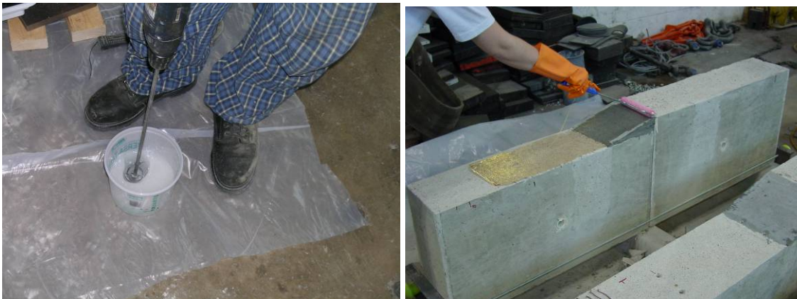
Figure 3-35 Mixing epoxy and saturating concrete surface
