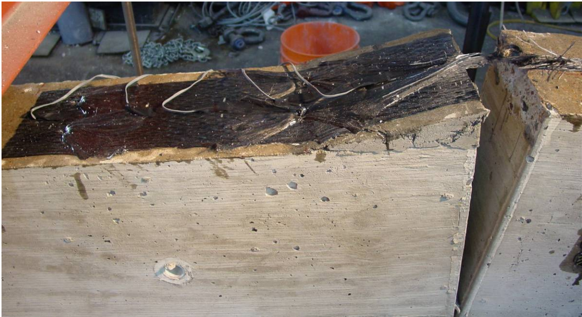
After Testing: Failure FRP fracture in column bundle, insufficient saturation
