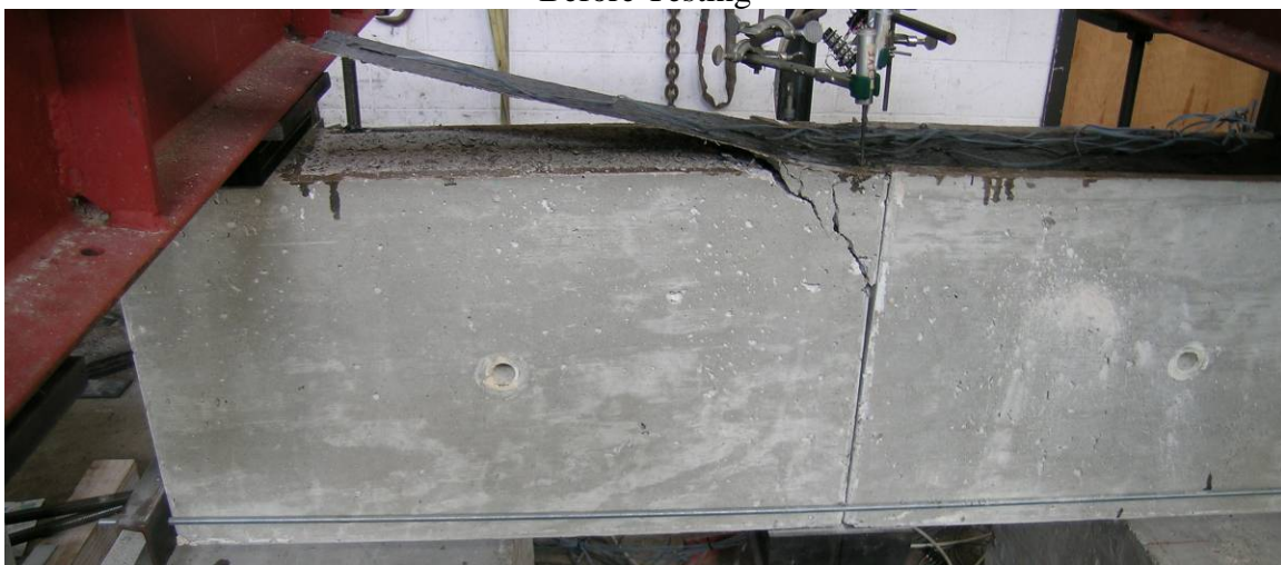
After Testing: Failure by corner crack and debonding
