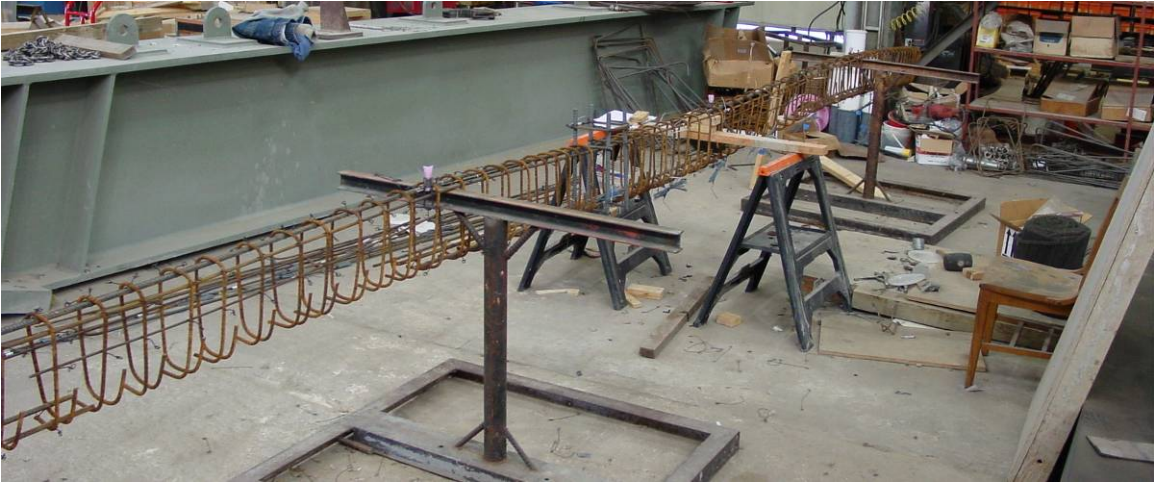
Reinforcement tying
