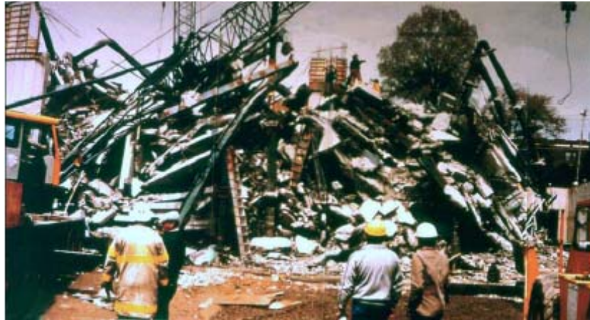
Figure 2-6 L'Ambiance Plaza collapse [NIST, 2007]
