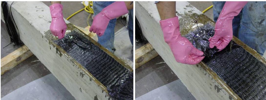
Figure 3-40 Inserting anchor and fanning ends of anchor over CFRP sheet
