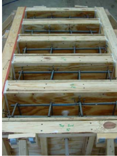
Figure 4-5 Concrete block formwork and rebar
