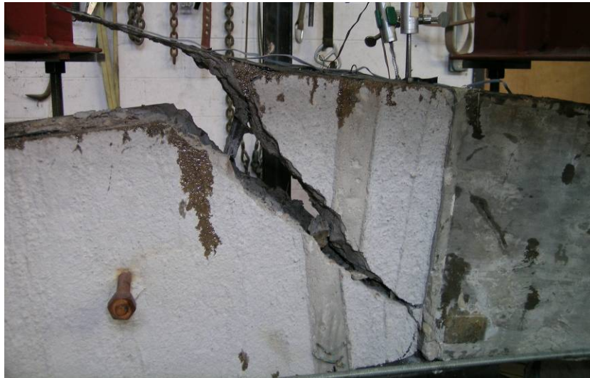
Figure 4-23 Failure by shear in concrete block (00-4g1)
