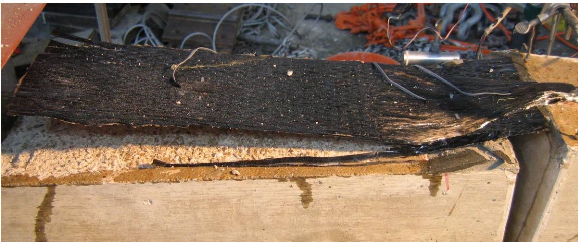
After Testing: Failure by debonding
