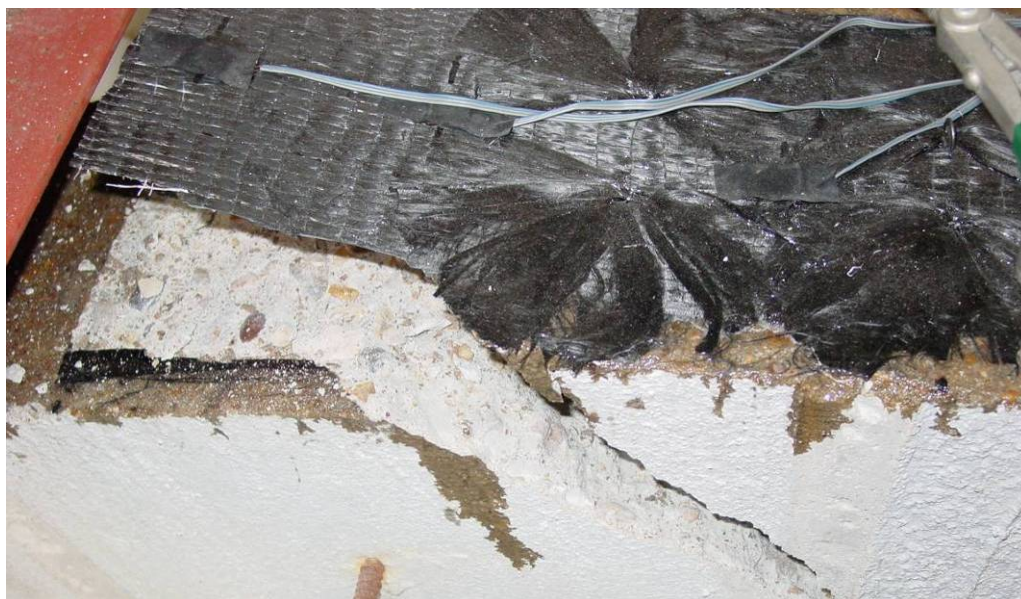
After Testing: Failure by shear in concrete block
