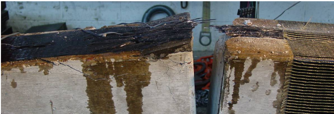
Figure 4-31 Failure of 41-6s1 with 1" height difference
