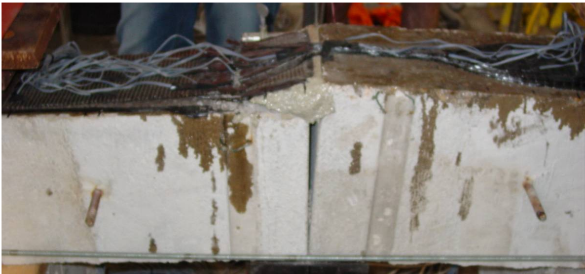
After Testing: Failure by Debonding
